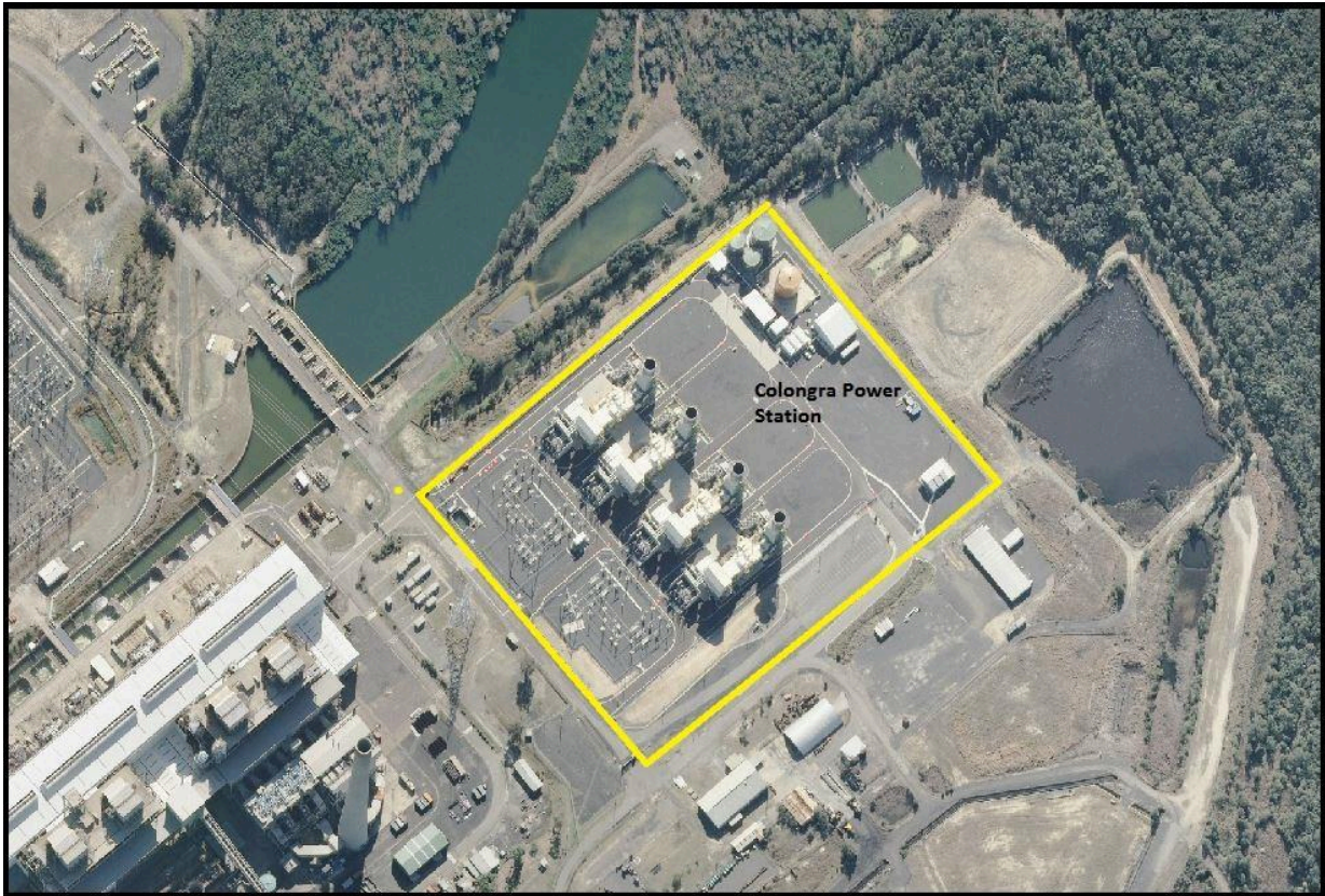
Figure 1 Colongra Power Station premises boundary for this AEMR
