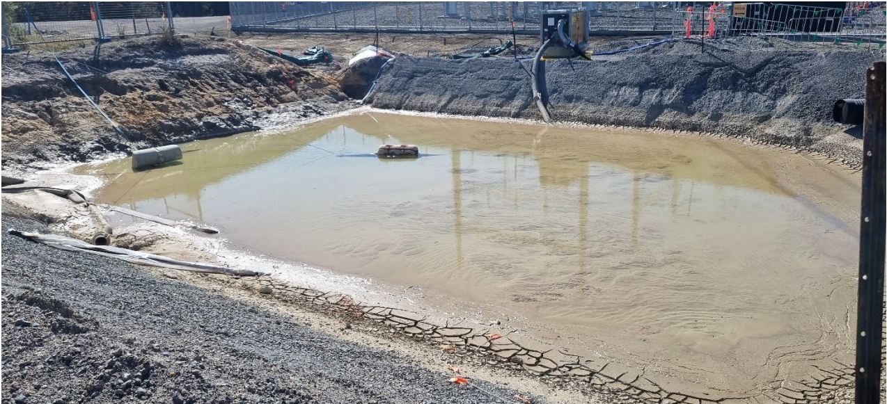
Photograph 5 - Area 1 Retention Basin
