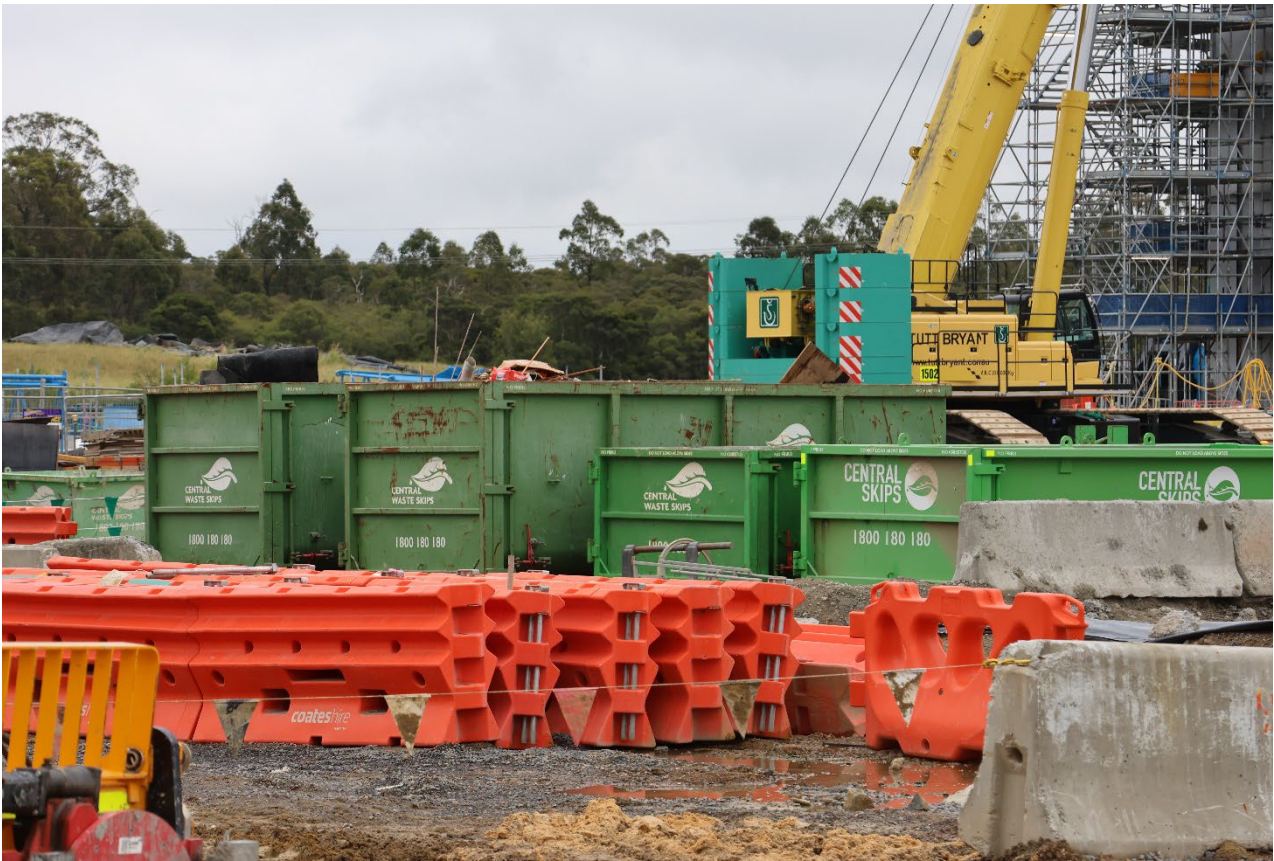
Photograph 7 - Construction Waste Storage
