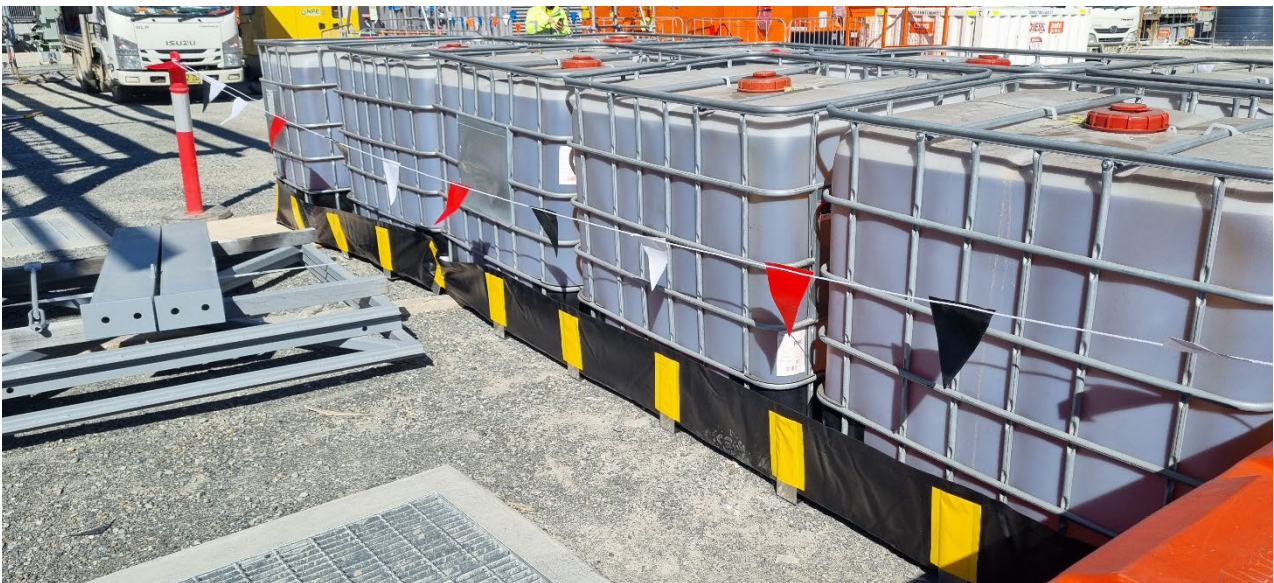
Photograph 2 - Temporary Bunding for Hazardous Chemicals Storage
