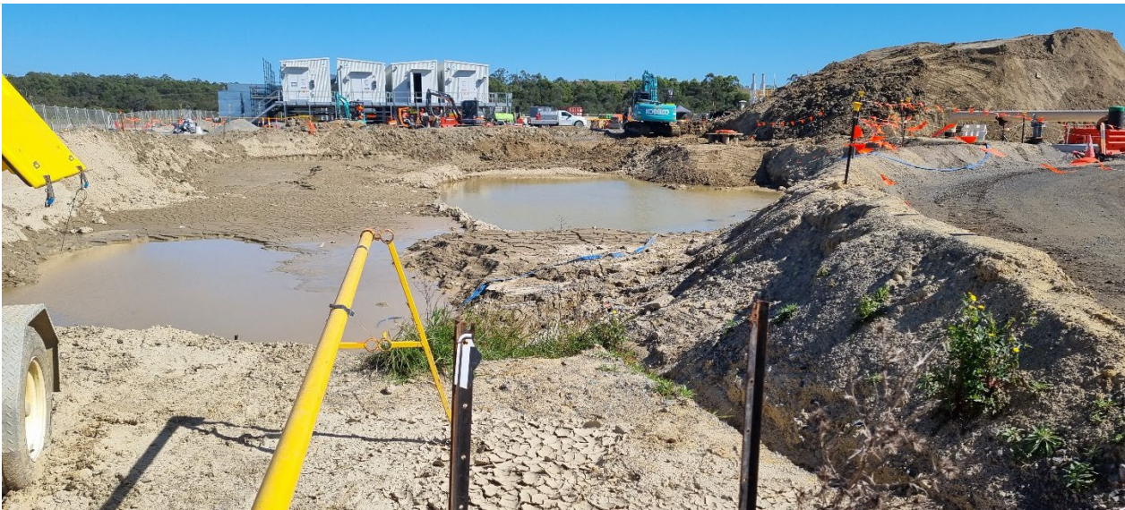
Photograph 4 - Area 2 Retention Basin
